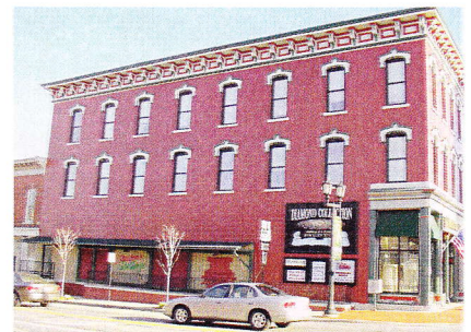
Painted masonry with historic color scheme
