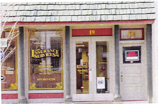
Historic entry and doors
