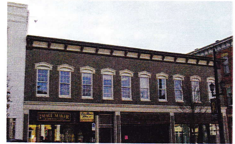
Original restored upper floor windows
