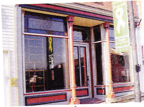
Restored wood trim storefront
