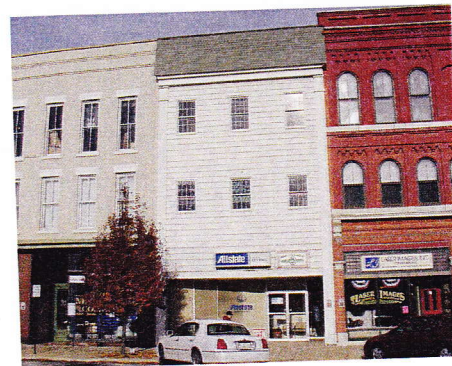
Restored wood facade
