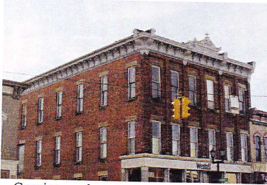
Cornice used as parapet
