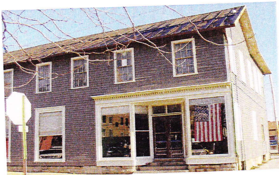
Restored wood facade
