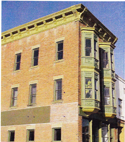
Original restored upper floor windows
