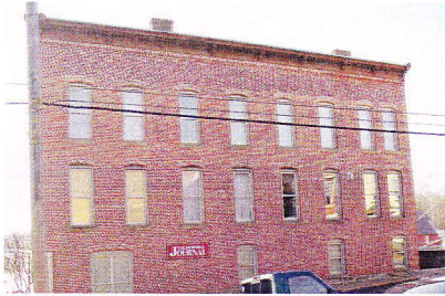
Restored original masonry & stone
